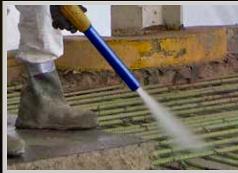
Concrete Repair & Restoration
